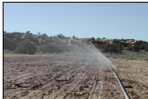
BP Americas Florence K5M showing sprinklers running, August 2003
