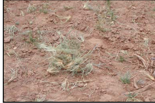
Williams Production Pipeline right-of-way with clumps of Hy Crest Crested Wheatgrass pulled out of soil, July 2003
