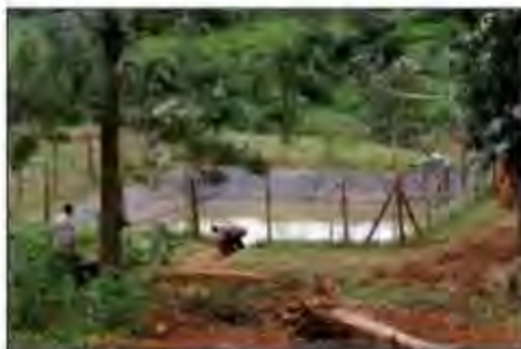
Rainwater harvesting collection pond in Rwanda
